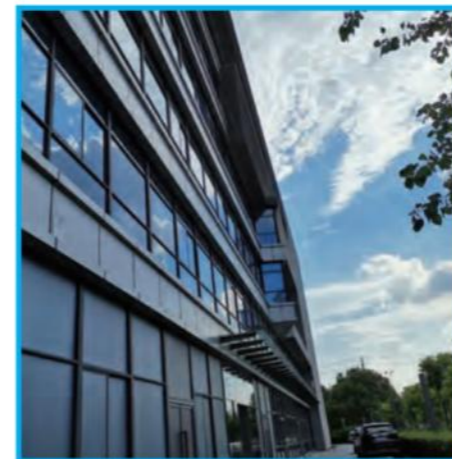
Shanghai Sales & Service Center
